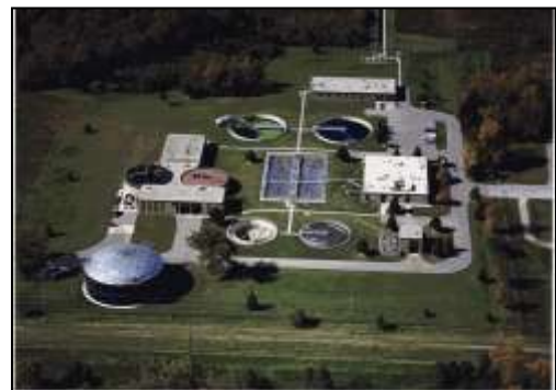
Oconomowoc Wastewater Facility
